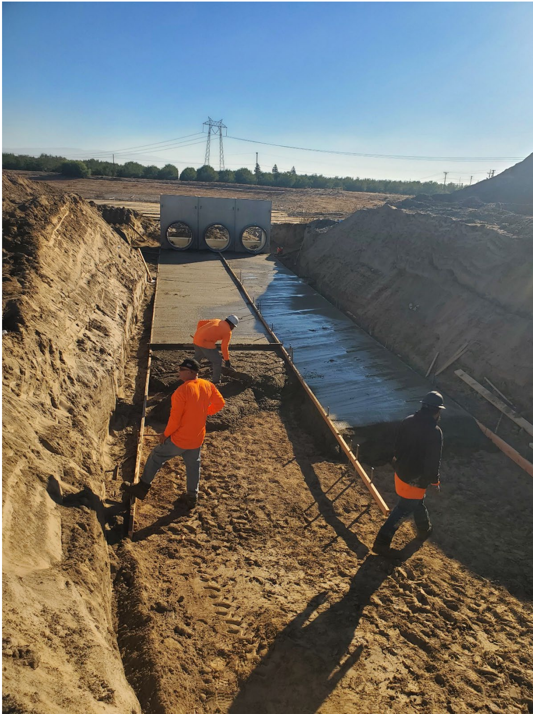
Placing Slurry Bedding
