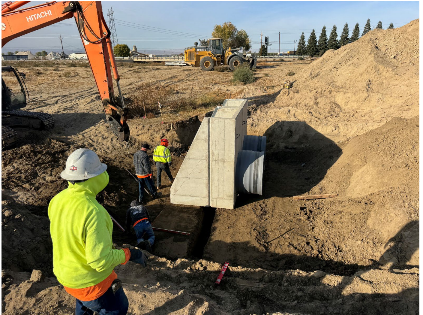
Placing Turnout Structures
