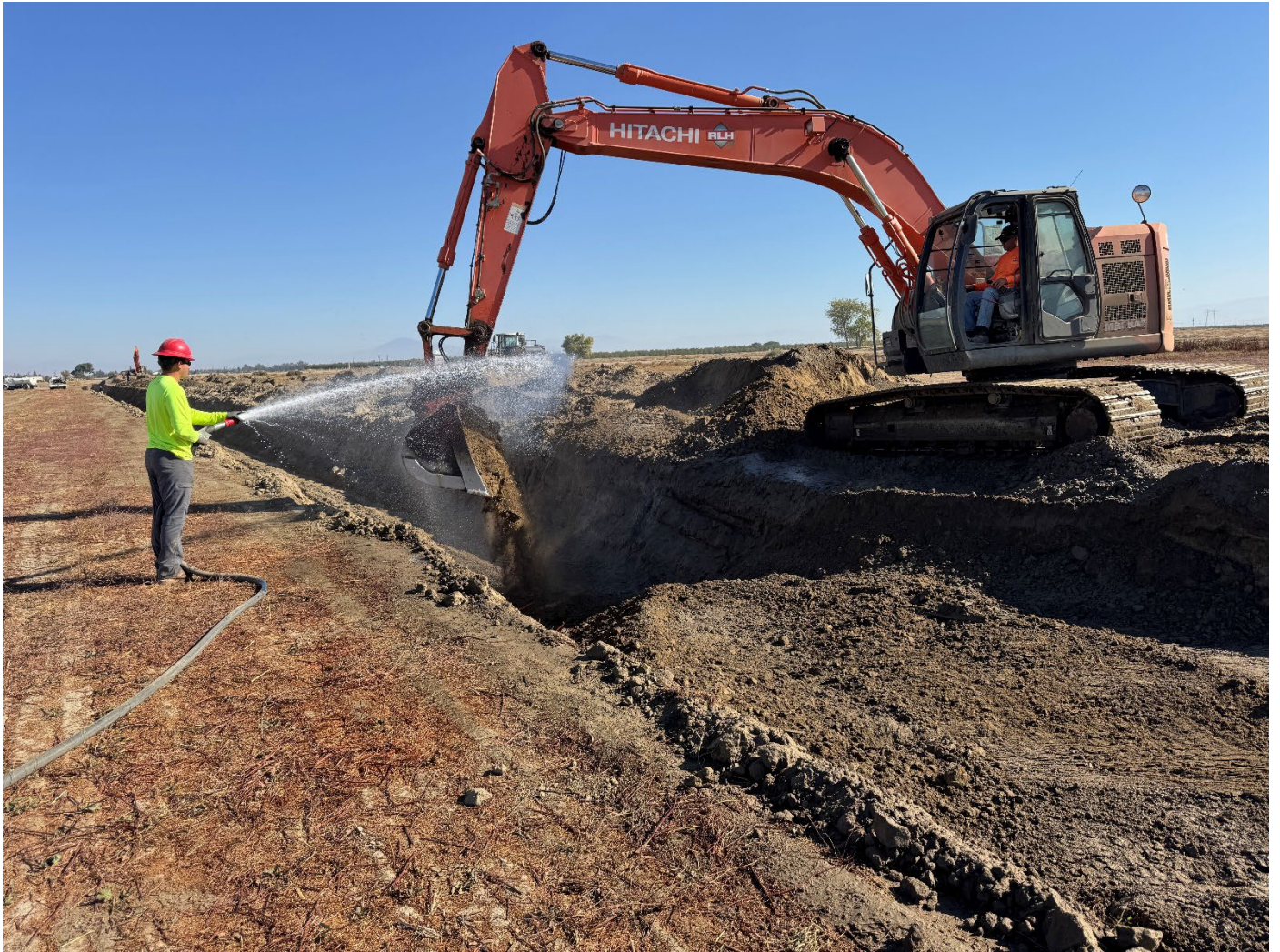
Backfilling above pipe around STA 75+00
