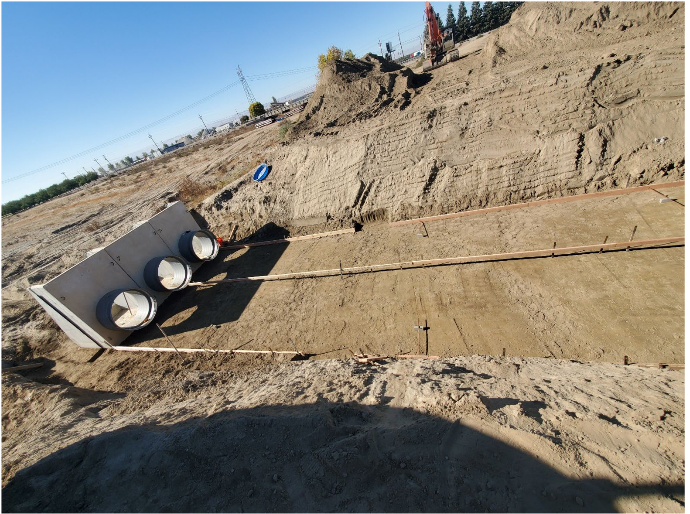
Line and Grade for Slurry Bedding
