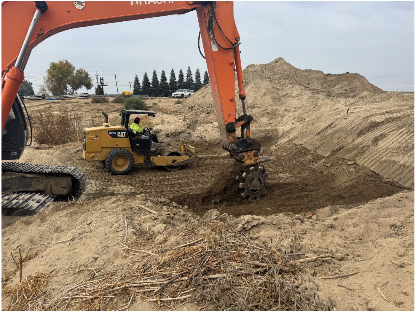
Compacting the Base for the Turnout Structure
