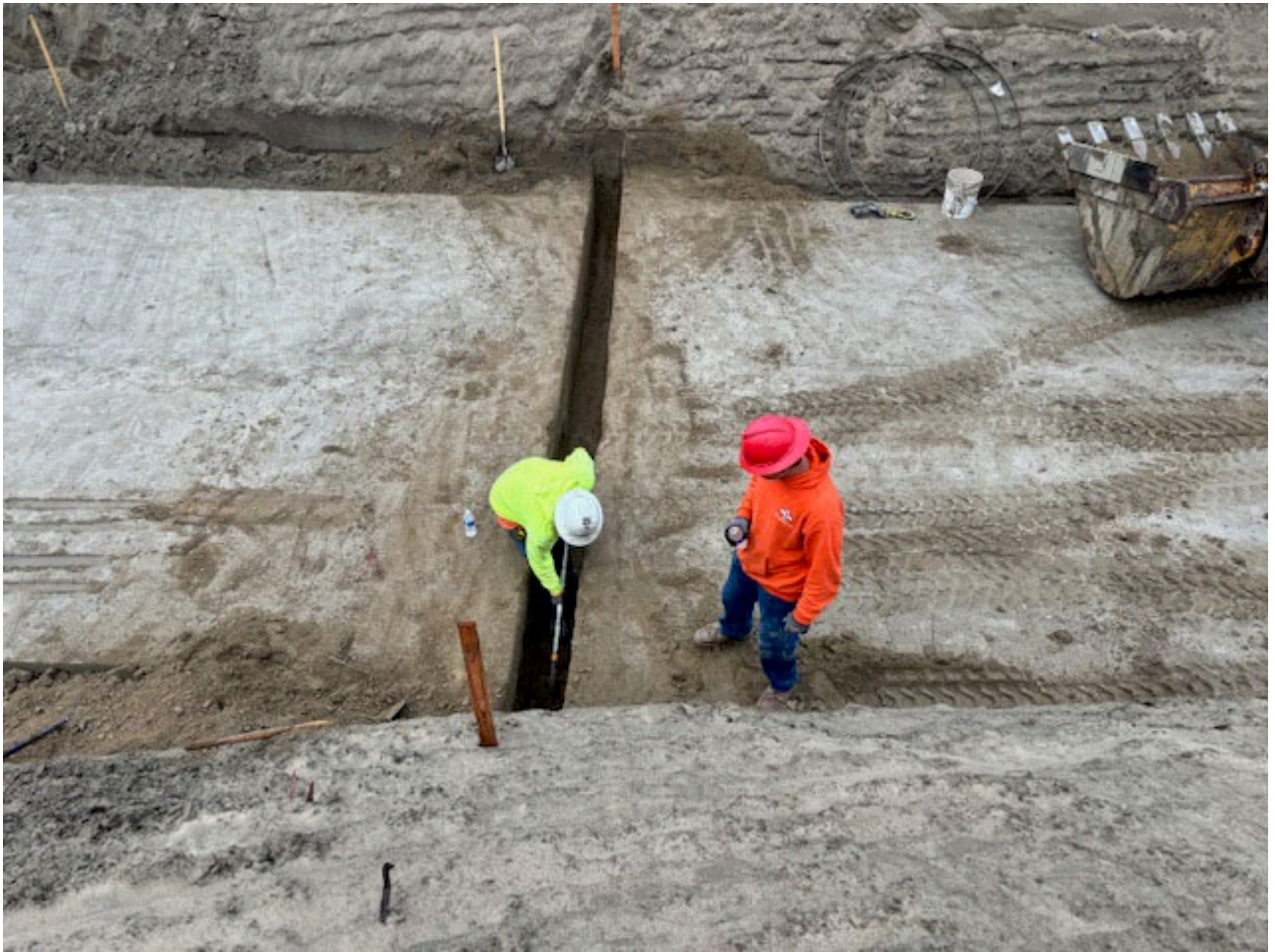
Excavating for Cutoff Collar
