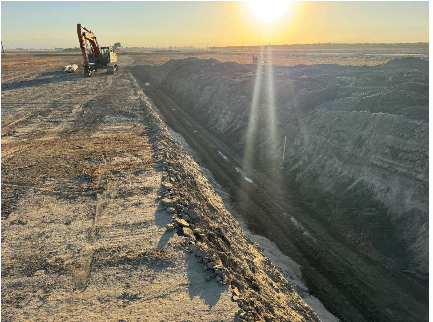
Soil Compacted at Top of Pipe Near STA 86+00, Facing Easterly
