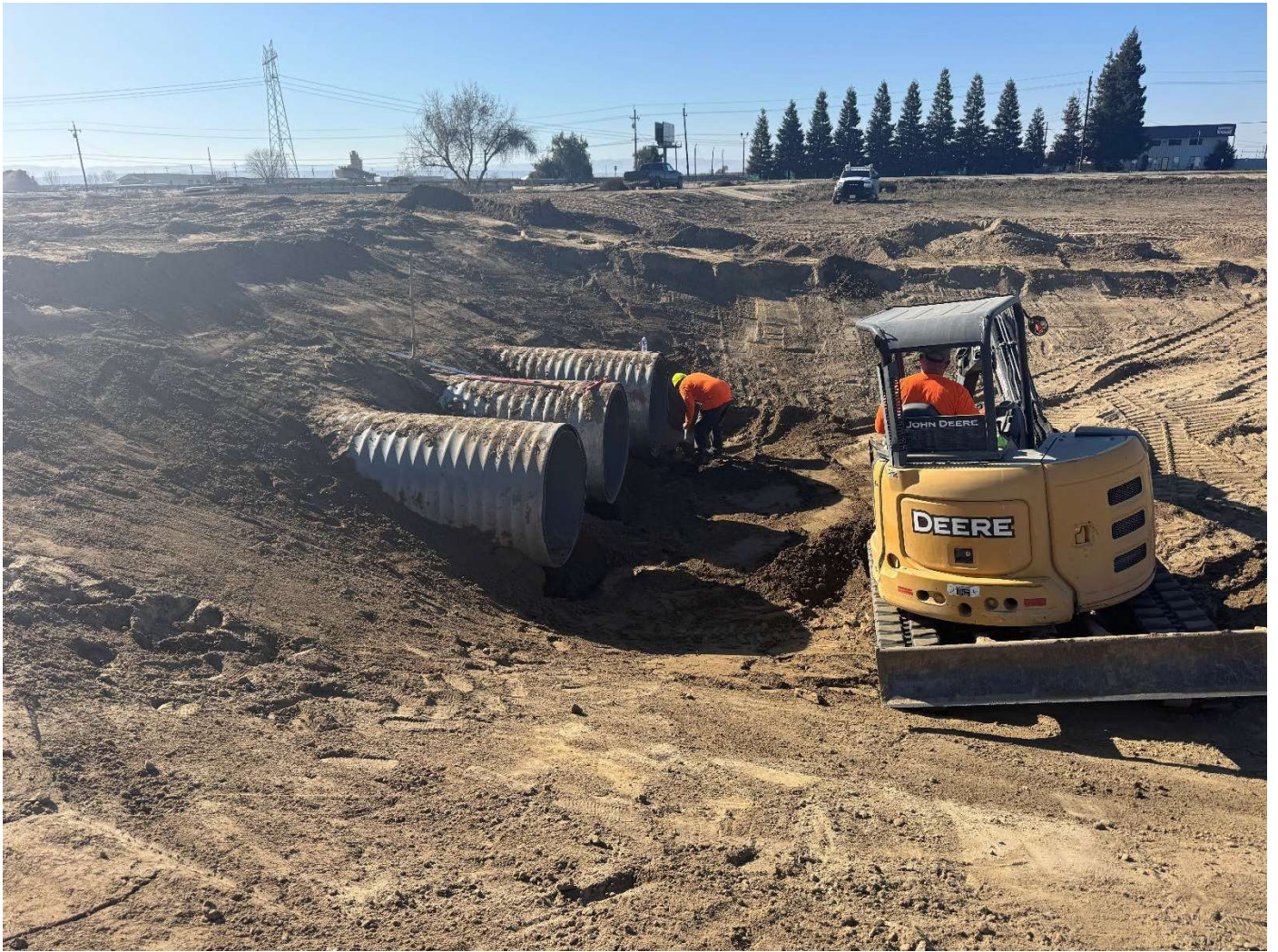
Grading for Outlet Channel from Goose Lake Turnout
