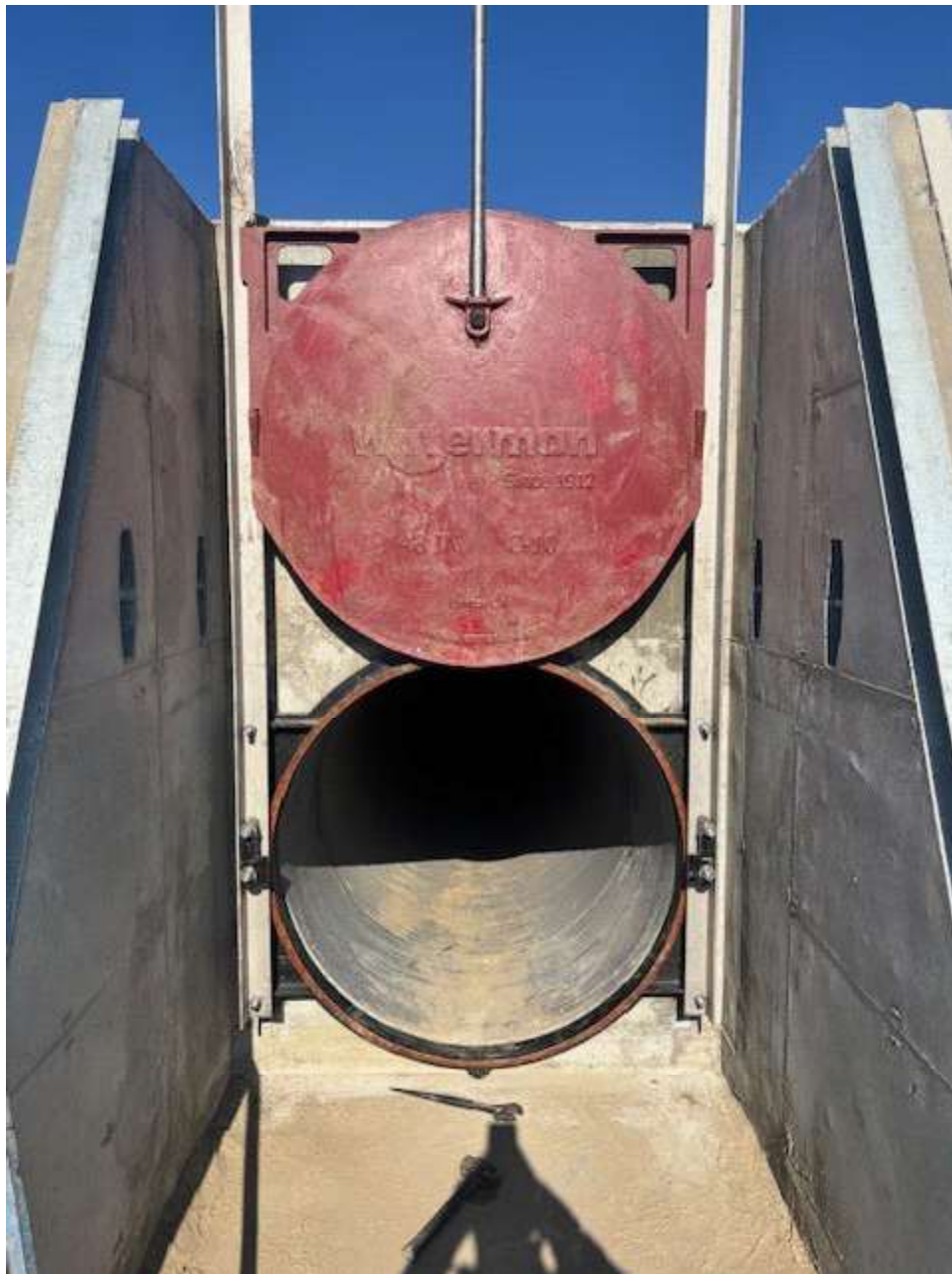
Slide Gate Installation
