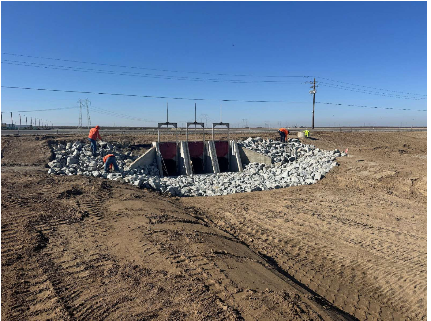
Rip-Rap Placement at West Enos Turnout
