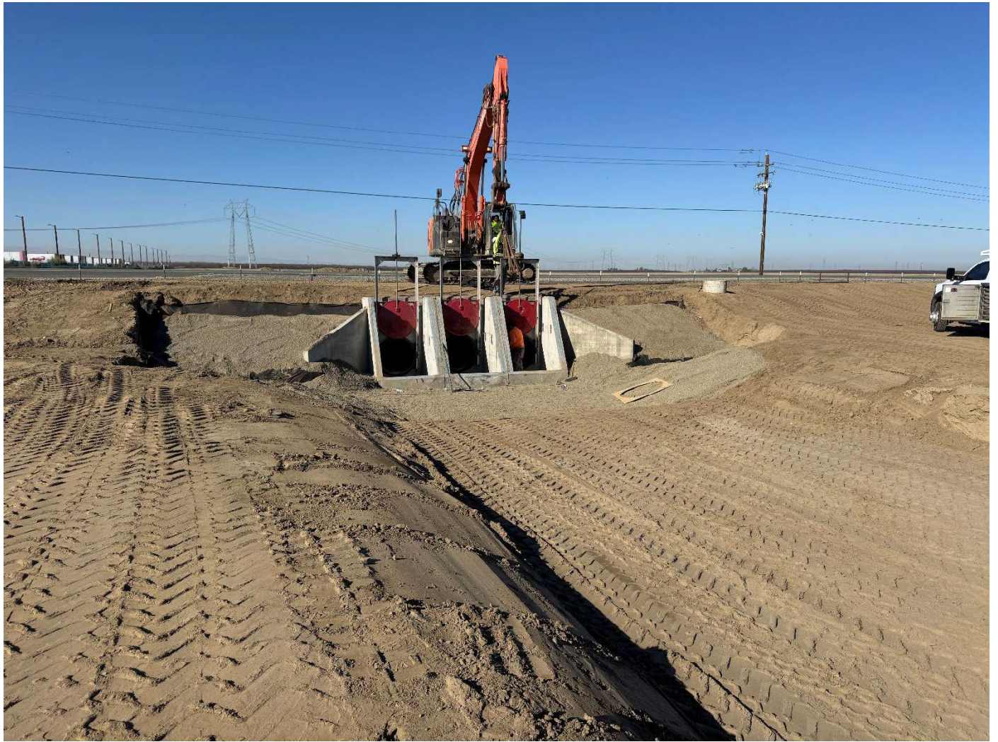
Finishing Installation of Slide Gates
