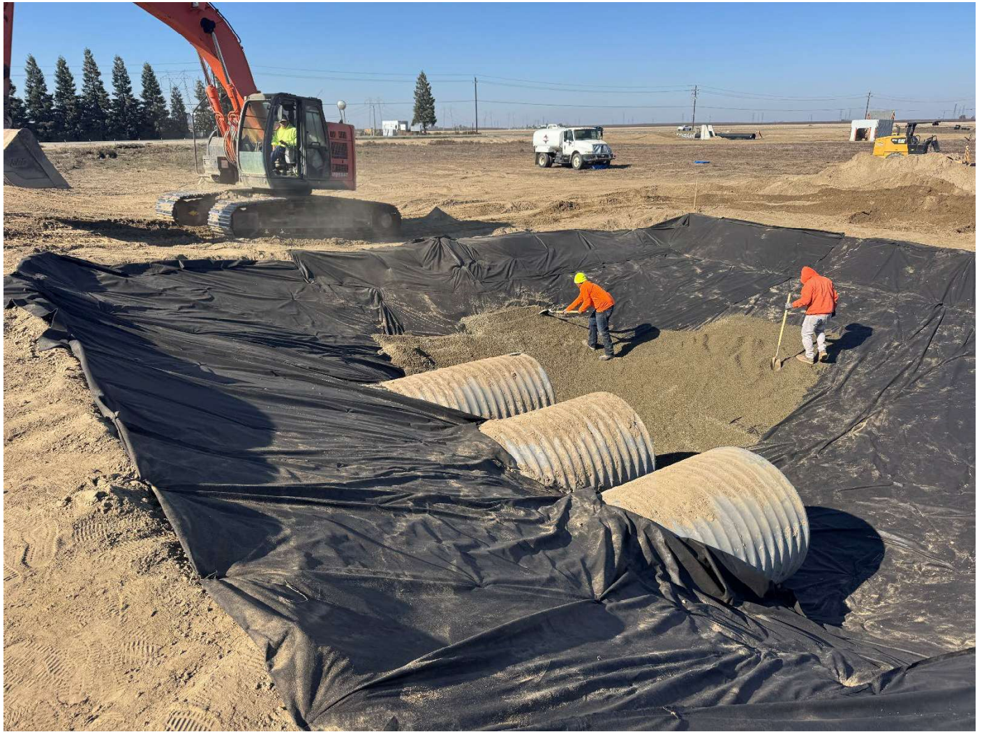
Spreading Pea Gravel on Outlet Channel of Goose Lake Slough Turnout
