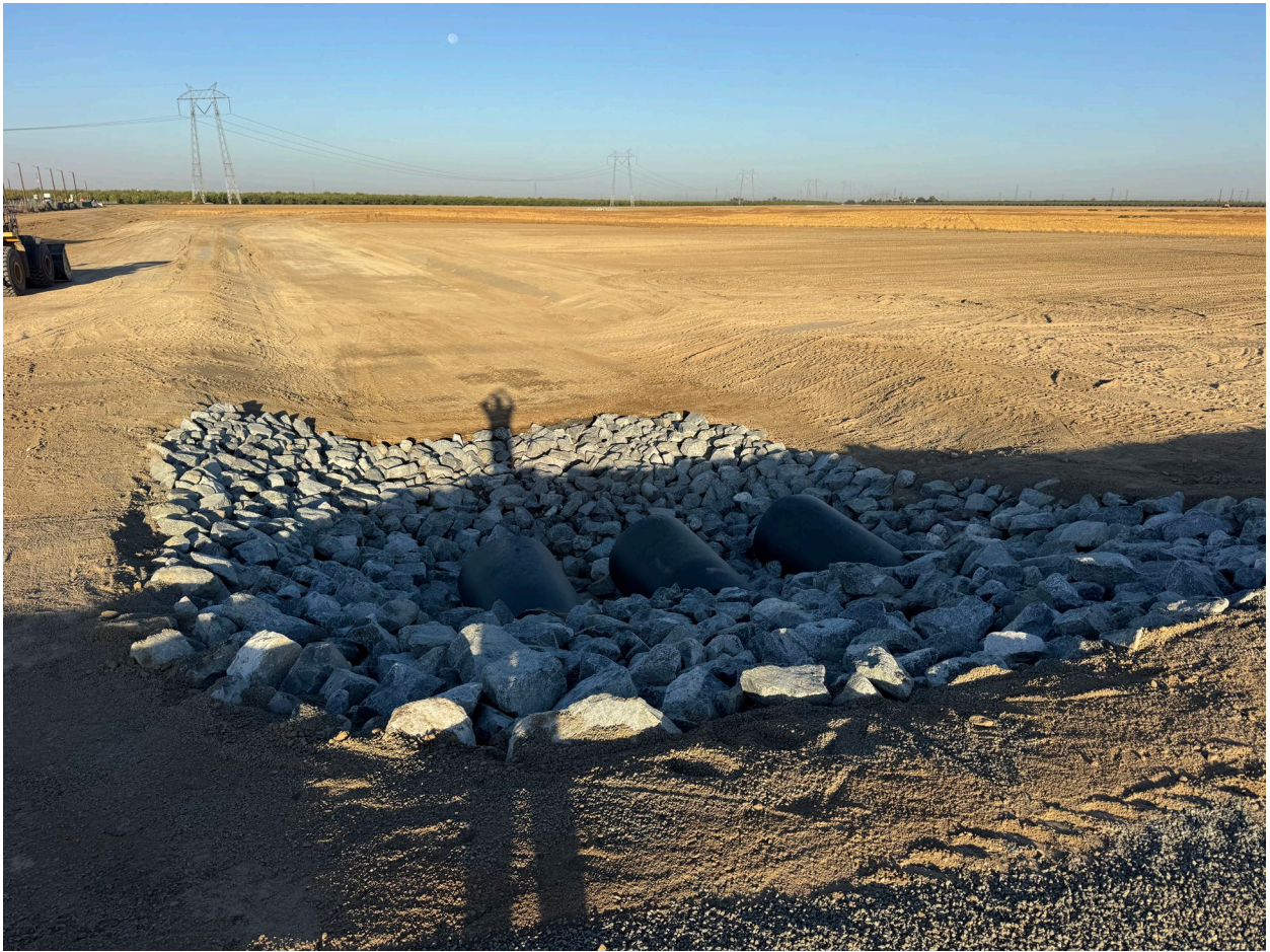
West Enos Crossing Outlet Rip-Rap
