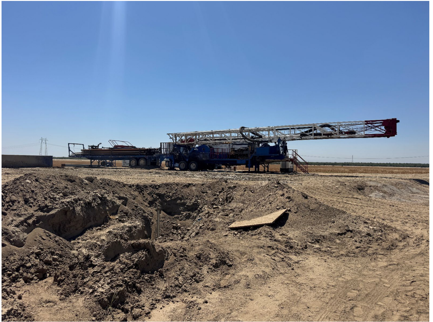
Removing Rig from the Site
