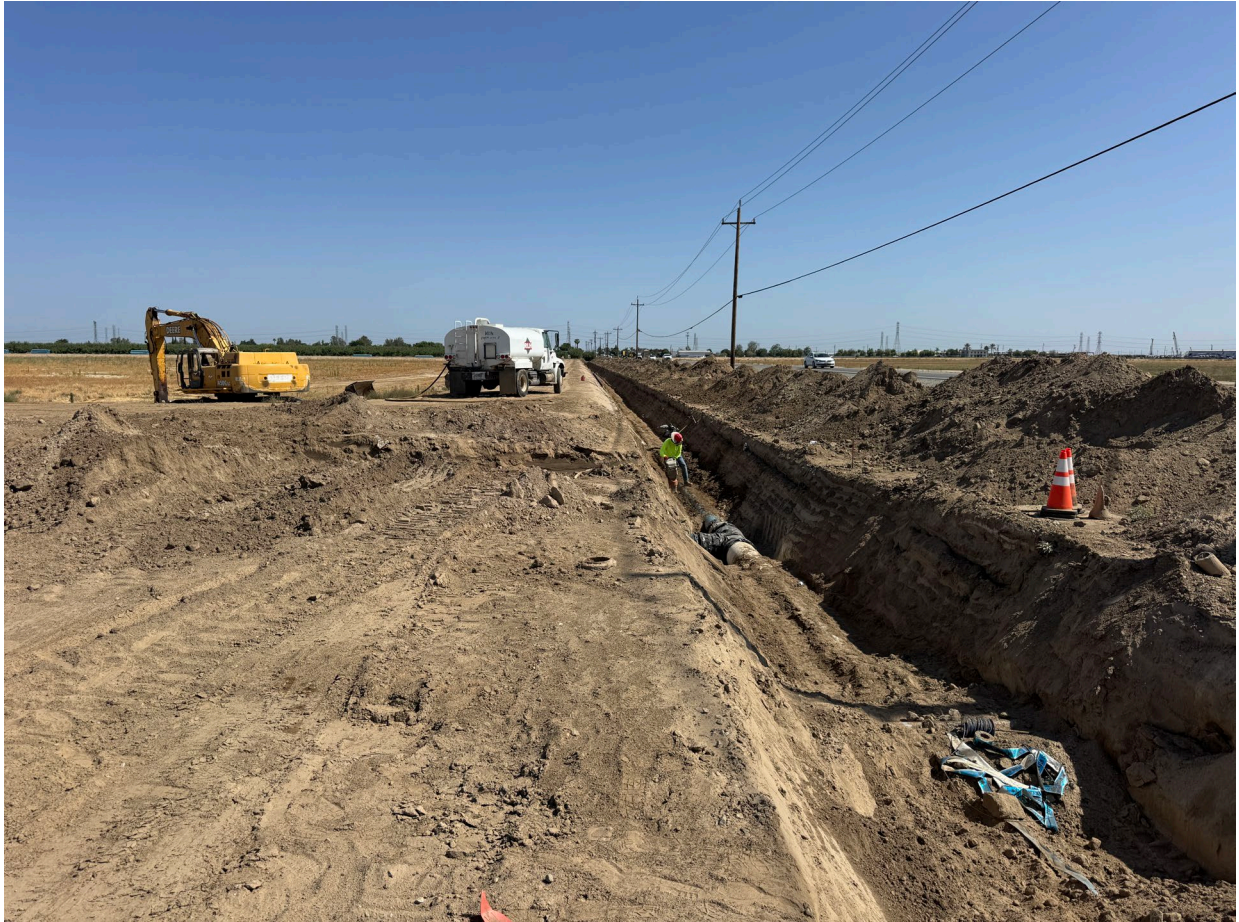
Pipeline Installation on West Side of Enos Lane
