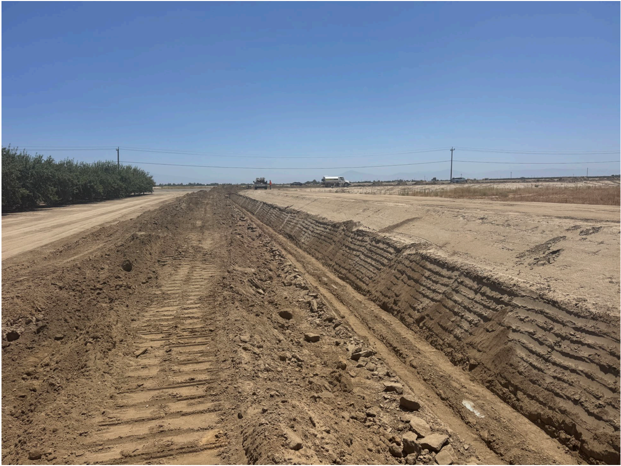
Pipeline Installation on North Side of West Enos Recharge Facility
