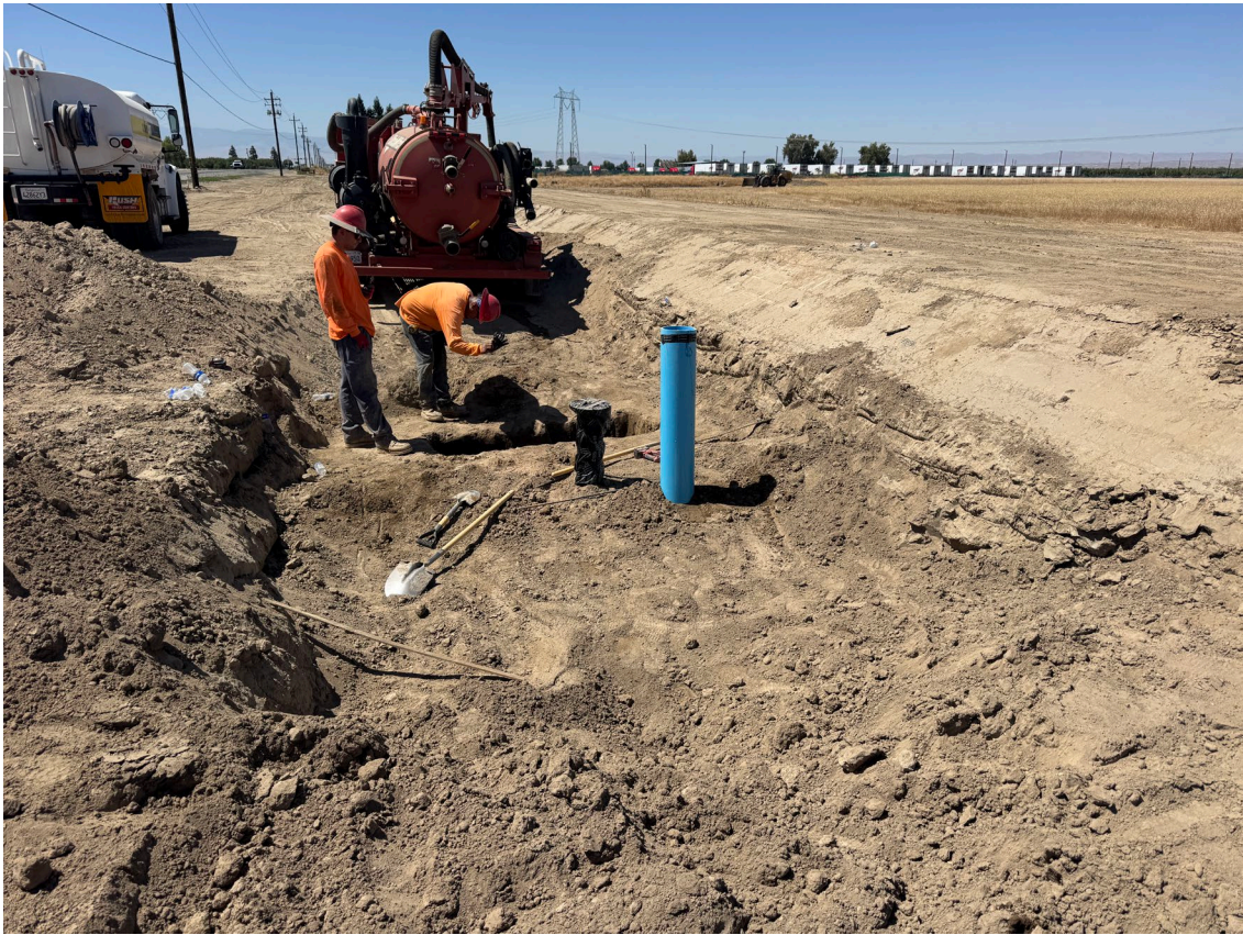
Installation of Water Supply Connection on West Side of Enos Lane
