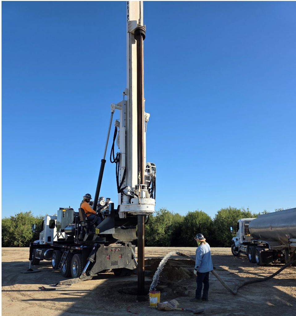
Conductor Casing Drilling
