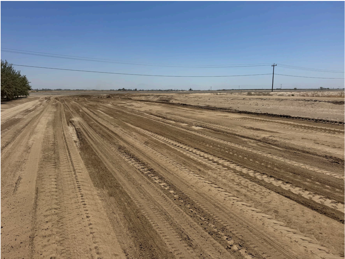
Fine Grading of Pipeline Alignment
