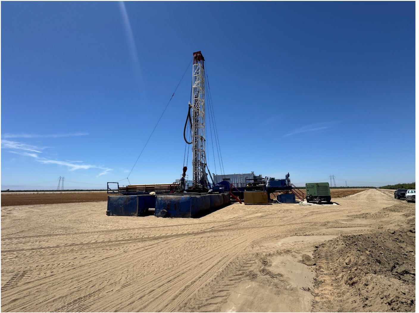
BW&P Mobilizing to West Enos Well #1 Site
