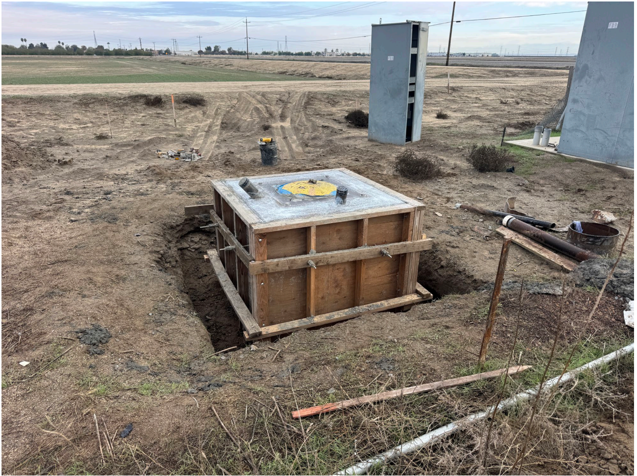
Well Foundation at WE-AG
