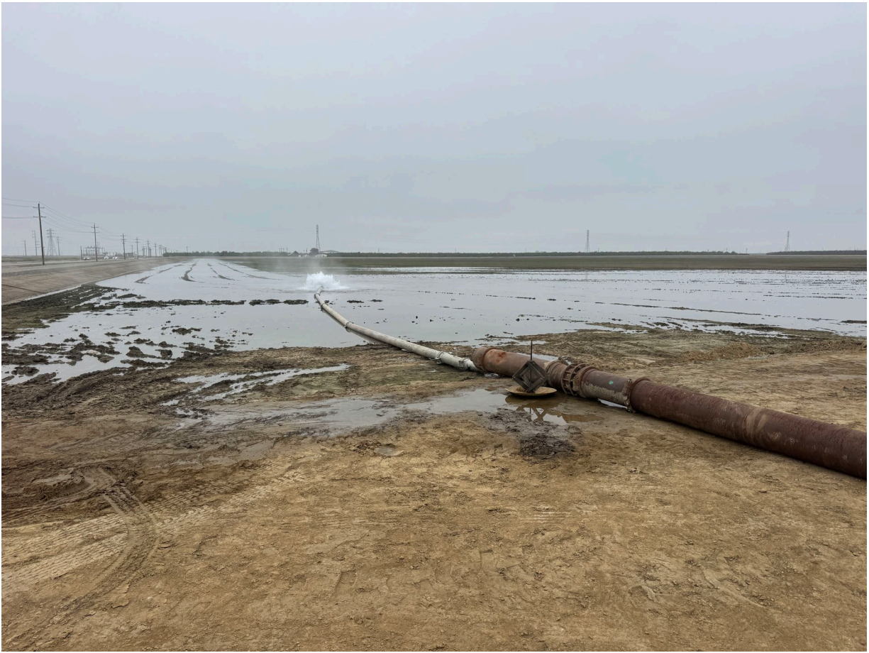
Well Development at SN-2
