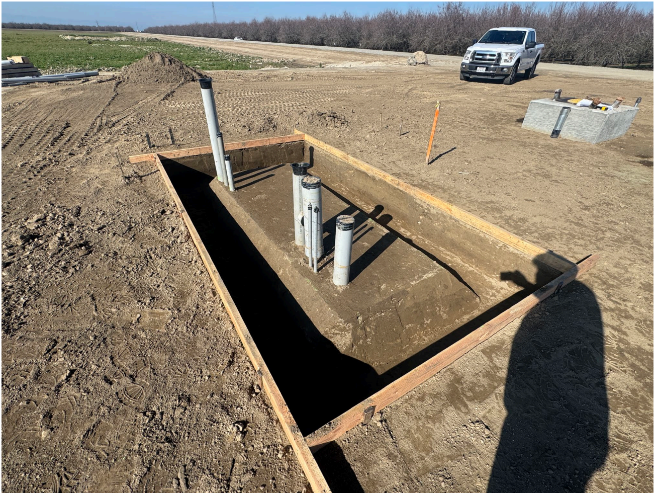
MCC Pad and Well Foundation at SN-2
