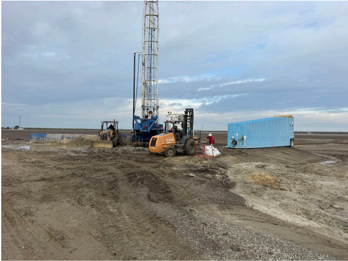
Drilling Rig Demobilization at SN-2
