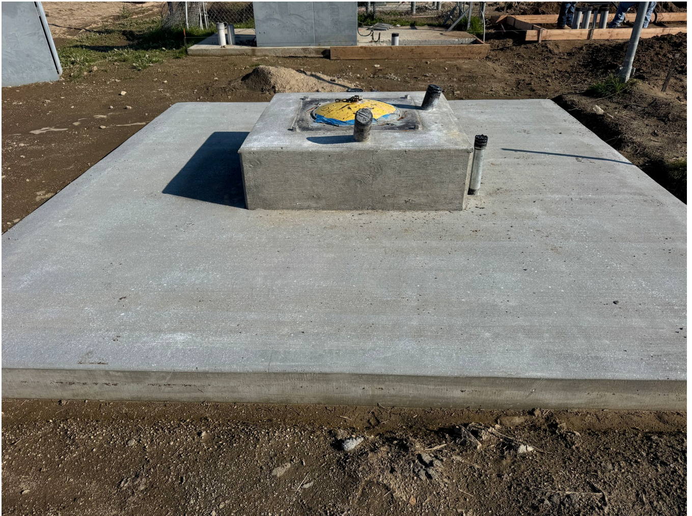
Well Foundation at WE-AG
